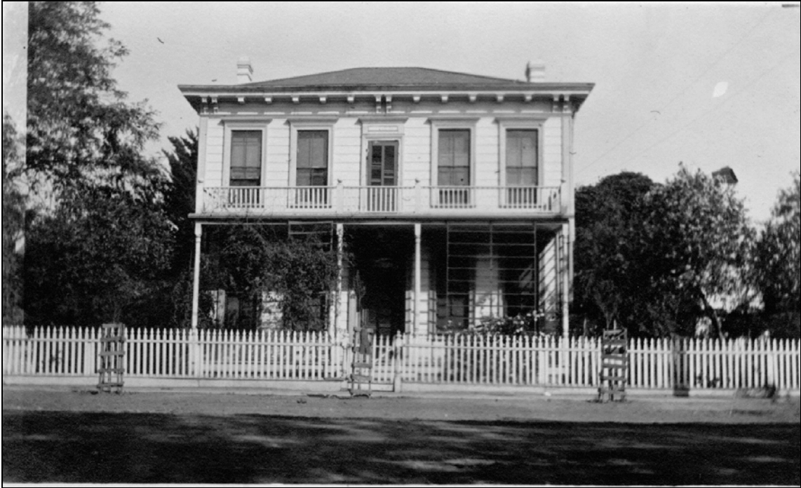
4.15. The Weber mansion at the northeast corner of Second and F, c. 1930. The George Augustus Weber family built this home c. 1880. Mr. Weber was a prosperous property owner and also owned and operated the Yolo Saloon and Billiard Parlor at Second and G Streets from virtually the founding of Davis until his death in 1914. The family of his daughter, Gertrude Weber Brinley, and her sister, Harriet Elisa Weber, lived in the home into the 1960s. Mr. Weber's grandson, John Weber Brinley, inherited the building, demolished it in 1963, and replaced with the structure we see in the next image. (John Weber Brinley.)
