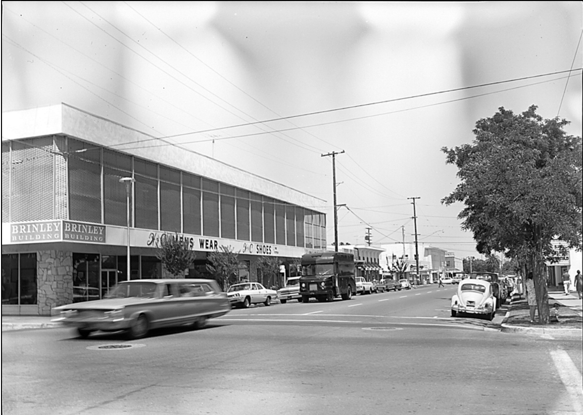
4.17. The Second Street 600s looking east, c. 1970. The building under construction in the previous image is now complete and, to the left, bears the name “The Brinley Building.” With the notable exception of the Terminal Hotel on the far eastern side of Second Street, the range of structures seen in this view have not changed substantially to this day. However, the overhead power lines are gone and the trees are much bigger. (Hattie Weber Museum of Davis.)
