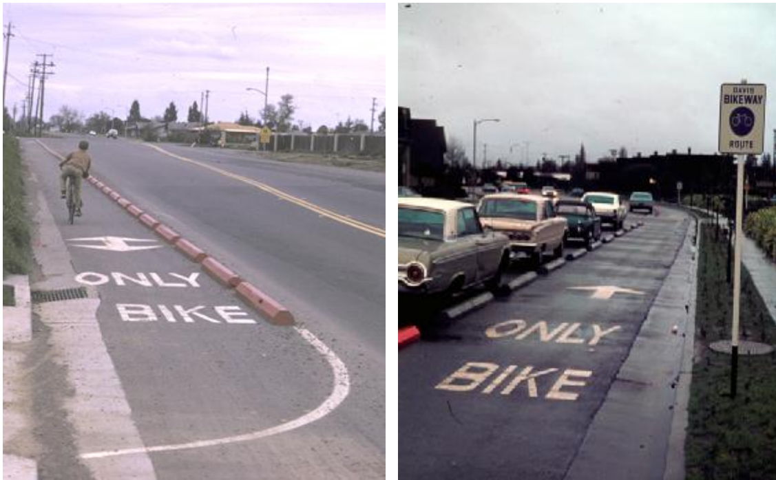
Figure 12 Bike lanes opened in Davis in 1967. Experimentation and refinement led to testing of different designs.
